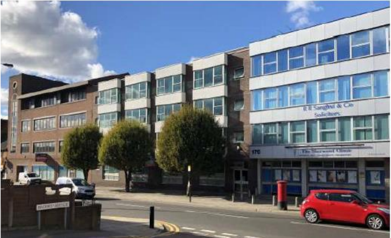
Front View (Above) & Rear View (Below)
